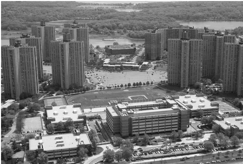
Figure 4. The Northeast Bronx Educational Park, including Harry S Truman High School and feeder schools, shares a modernist aesthetic and massive scale with surrounding Co-op City housing. Shown in this 2009 image, Truman is the large, mid-rise building at the center foreground, surrounded by four lower-rise elementary and intermediate schools, with apartment towers behind. (Photograph by David L. Roush, from Wikimedia Commons.)
